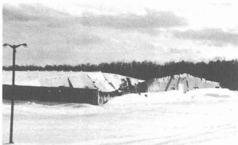
ROOF CAVES — The Feast building at Mount Pocono, Pa., suffered a disastrous cave-in Jan. 28 after snow and ice accumulated on its roof during a storm. The damage may mean no Feast at the Poconos in 1978. (See article, page 1.)
