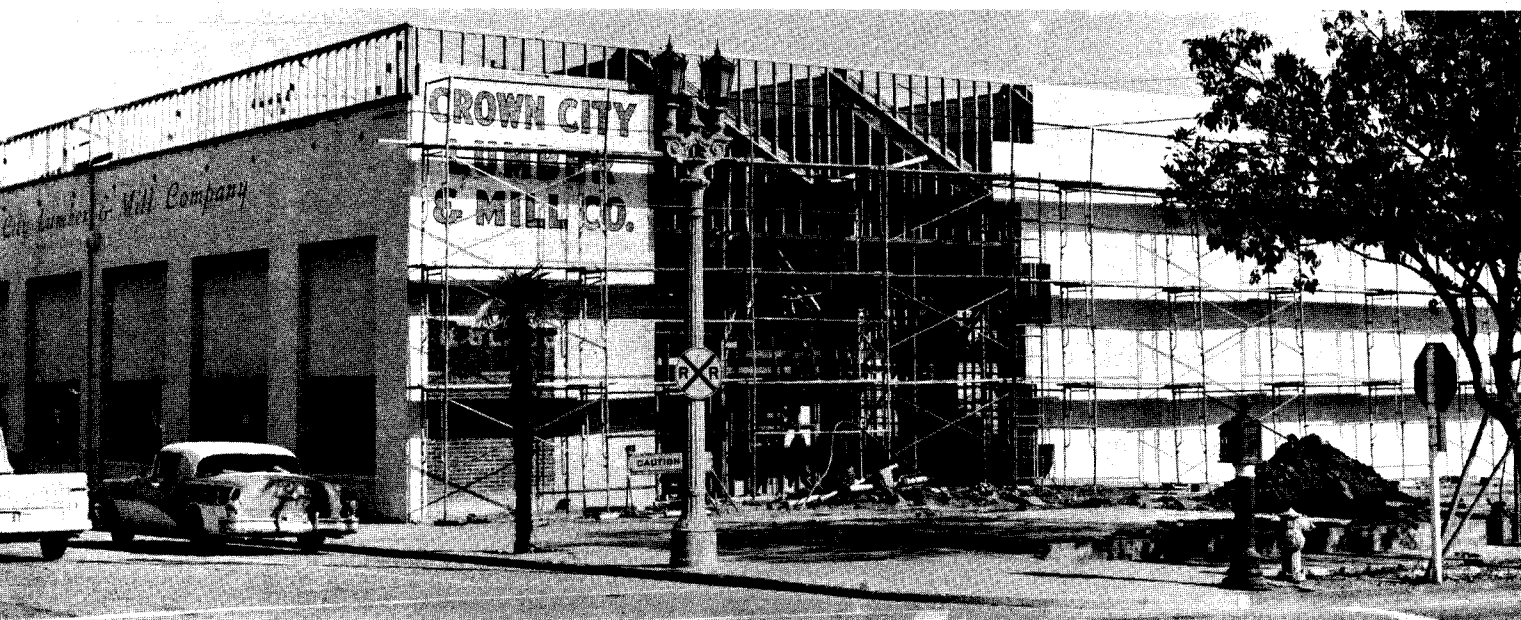
Below — Later the entire printing department was moved to the acquired Crown Lumber Company, shown in the process of being remodeled.
