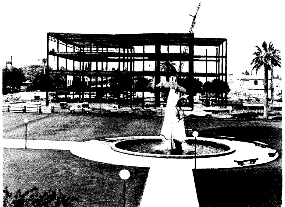
In February the steel girders were raised and in a few days the skeleton of the building began to take shape.
