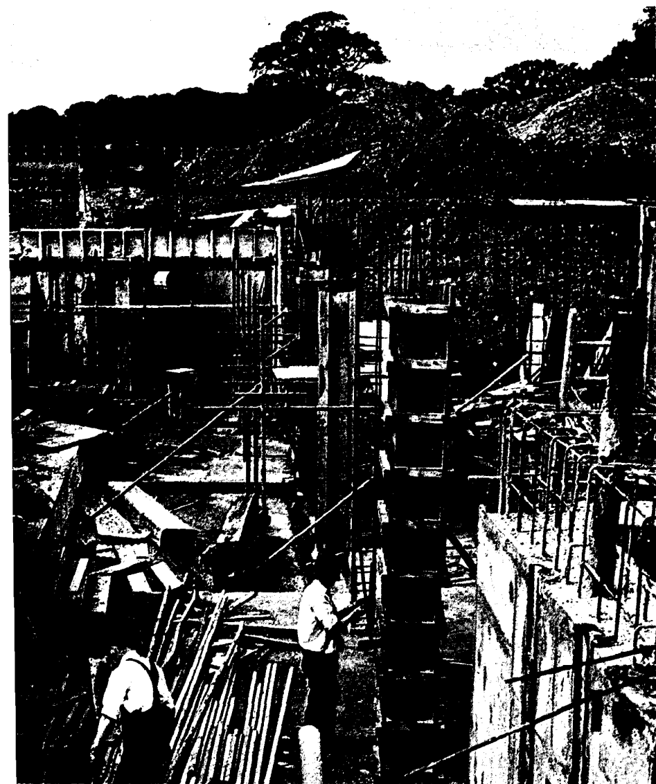
ABOVE —In the latter stages of construction the gymnasium begins to take shape. Notice the McAlpine construction firm's sign beside the scaffolding at the right. LEFT —Huge crane lifts steel girder cross beam toward its position in gym roof. CENTER —Complicated network of reinforcing steel rods insure structural strength —a factor unseen in the finished building.
