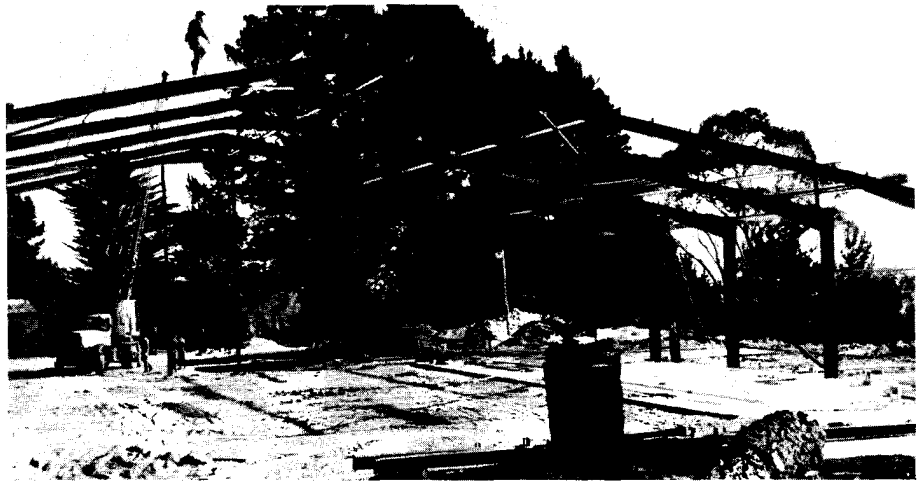
Here is a candid shot of a portion of the steel framework which will become the Tabernacle for the Festivals for the brethren in Australia. BELOW: An artist's conception of the finished Tabernacle.
