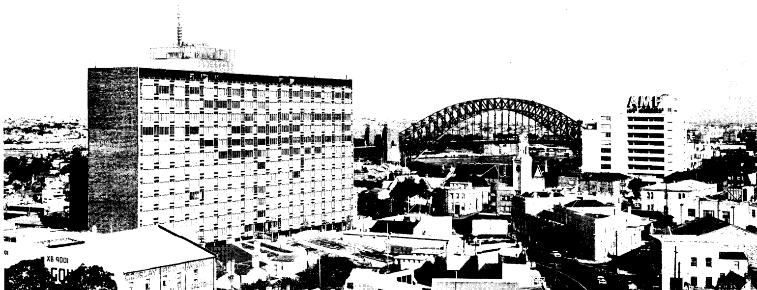
Offices of the Australian Work are located in this building.
